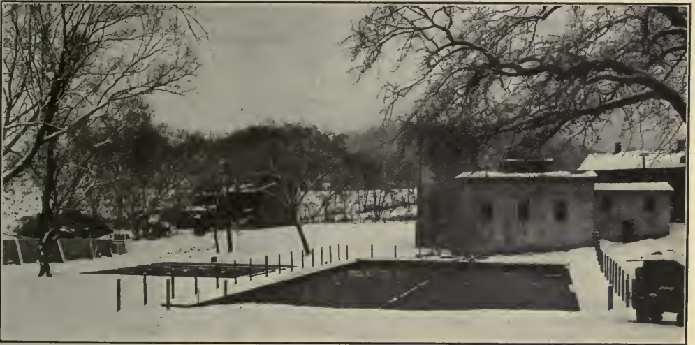
EXTERIOR OF THE PHILLIPSBURG, N. J., SEWAGE WORKS
